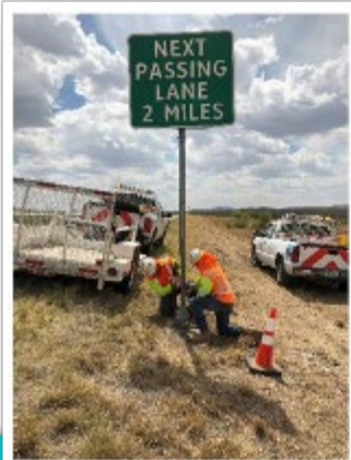
Passing lane signs installed
